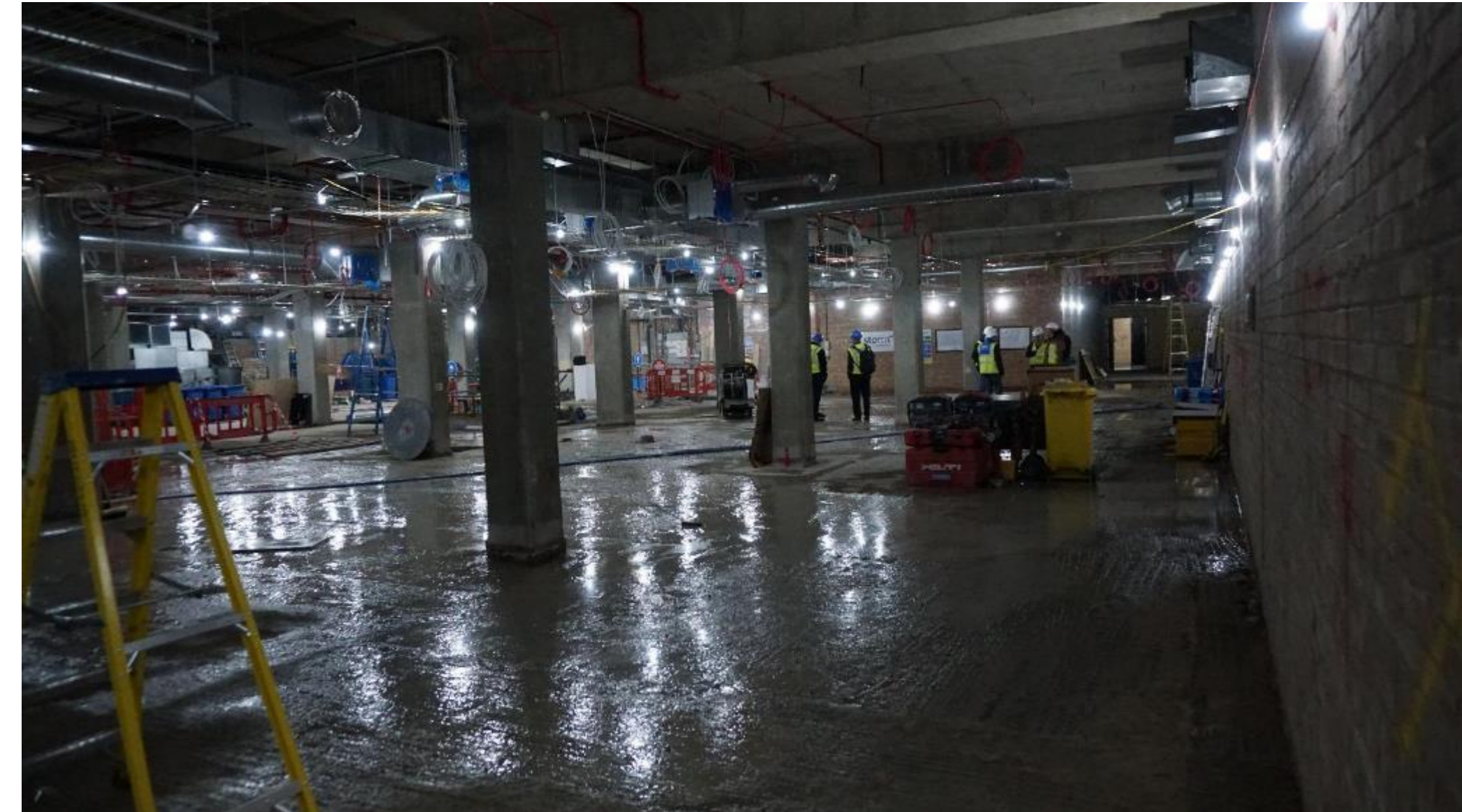
Construction in Progress
