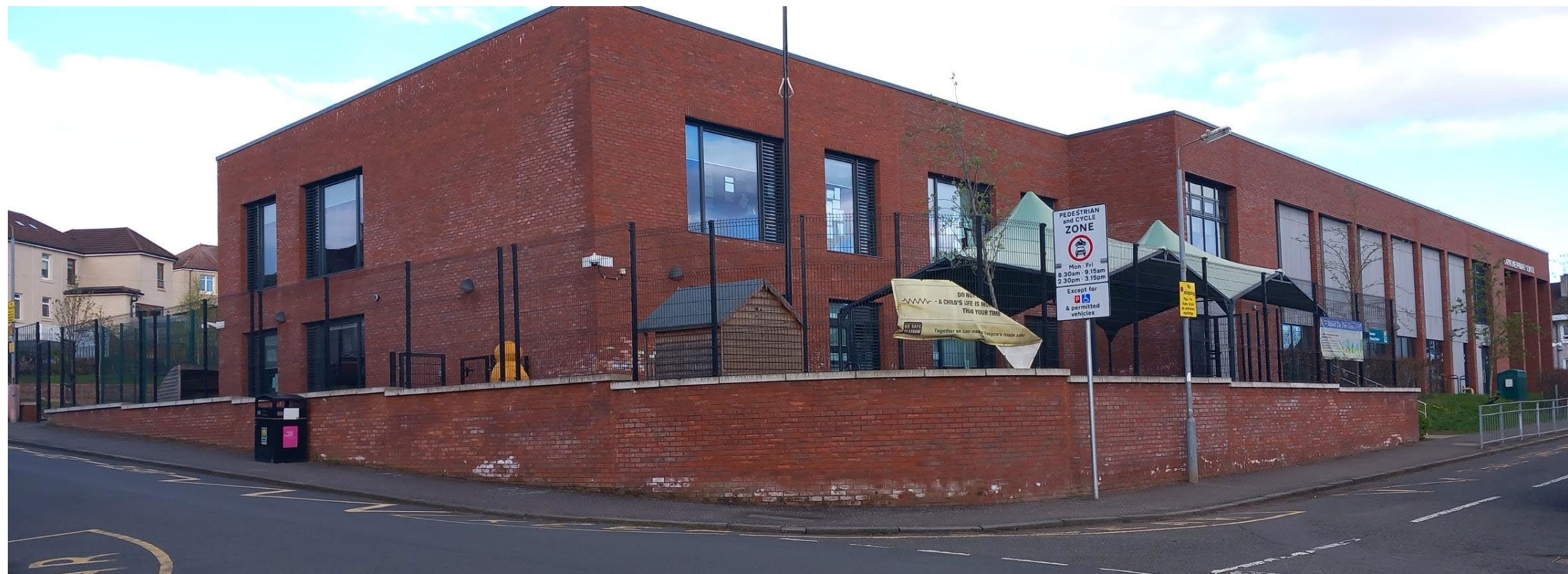
➤ Exterior of the extension:
